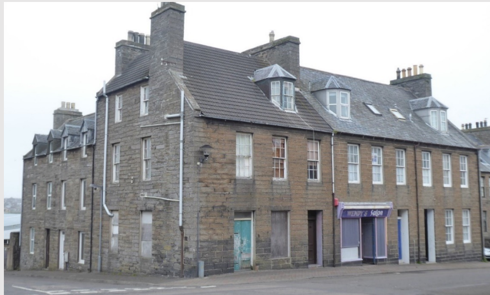
Historic buildings effected by inappropriate change
