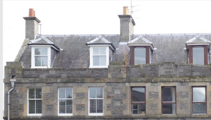
Inappropriate replacement windows
