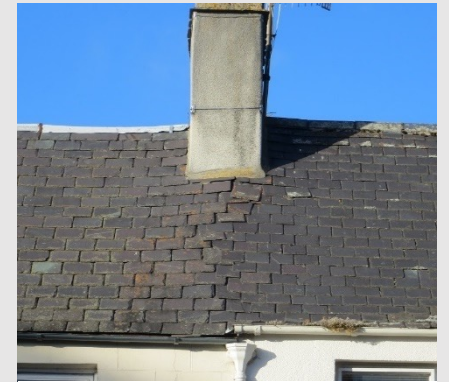
Stone copes removed
