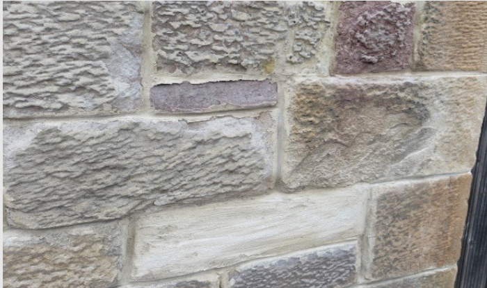
Cementitious mortar and plastic stone repair.
